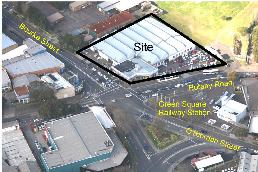
Figure 4: View toward the south-east illustrating Site at intersection of Bourke Street, Botany Road and O'Riordan Street
